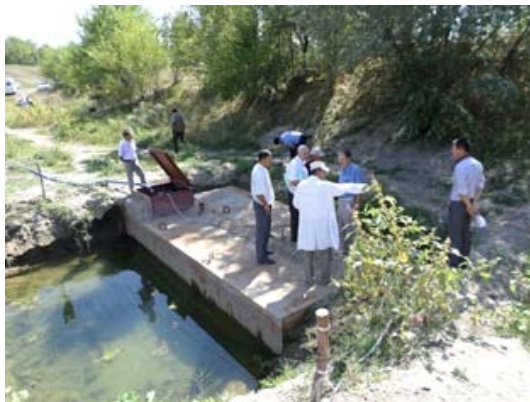
Fig. 1. Water intake system for drip irrigation
