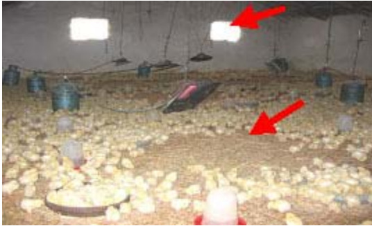
Plate 1: Breeding buildings were poorly ventilated and poorly heated
