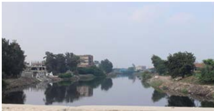
Photo. 1. Outfall of Belbies drain
