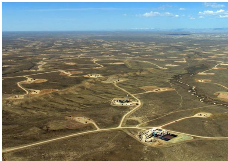
Fig. 5. Impact of exploration and production of shale gas on the landscape A view from the airplane to Jonah deposit, Wyoming, May, 2006. Photo: SkyTruth
